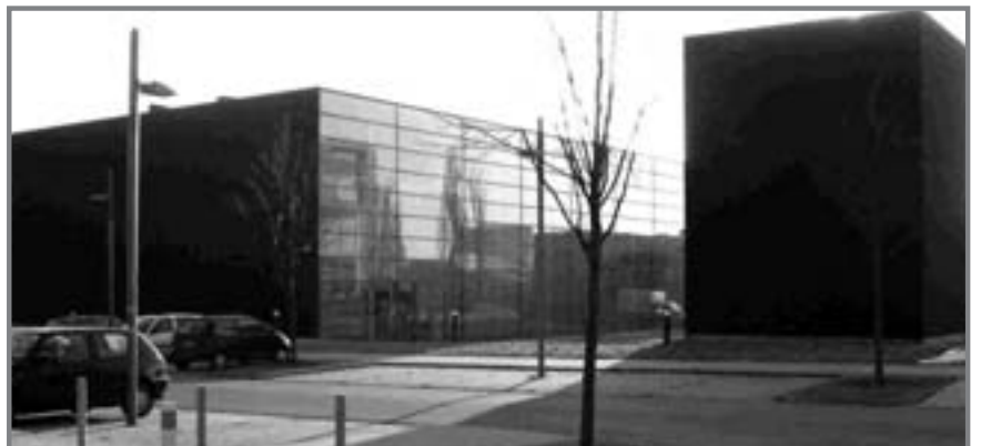
The Coda Audio Headquarters in Hannover, Germany
